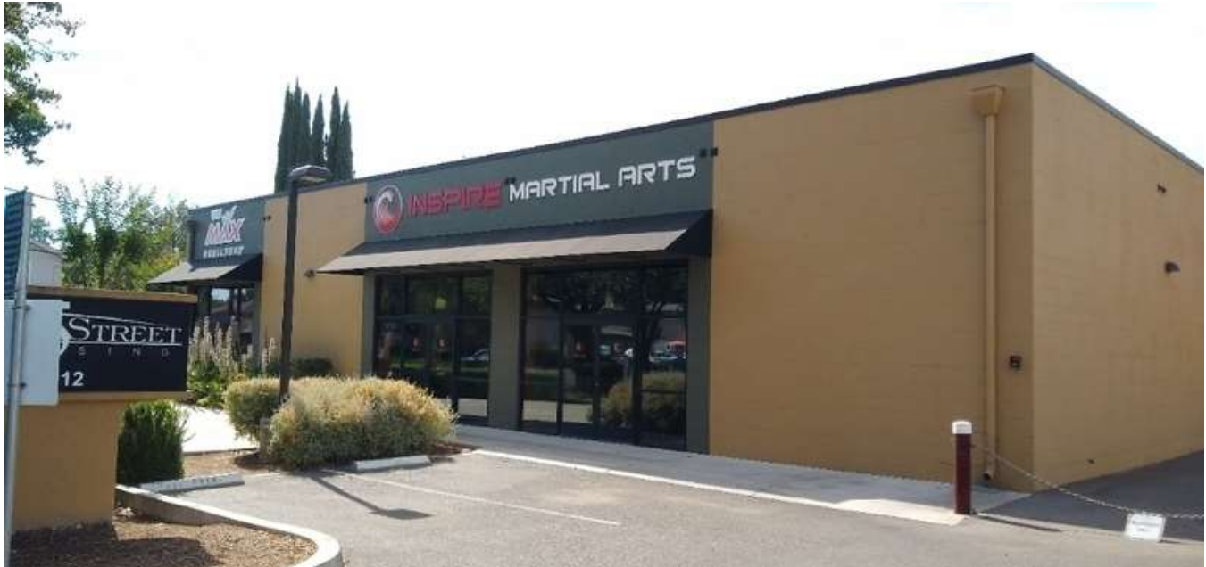
North (primary) façade, looking south. ESA, 2022.
